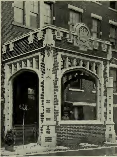
PORT COCHERE, BETH ISRAEL HOSPITAL, NEWARK, N. J. Terra cotta work executed by the New York Archi- tectural Terra Cotta Company. Nathan Myers, Architect.
